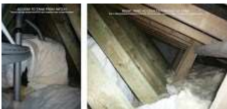
Roof access.jpg 145K
